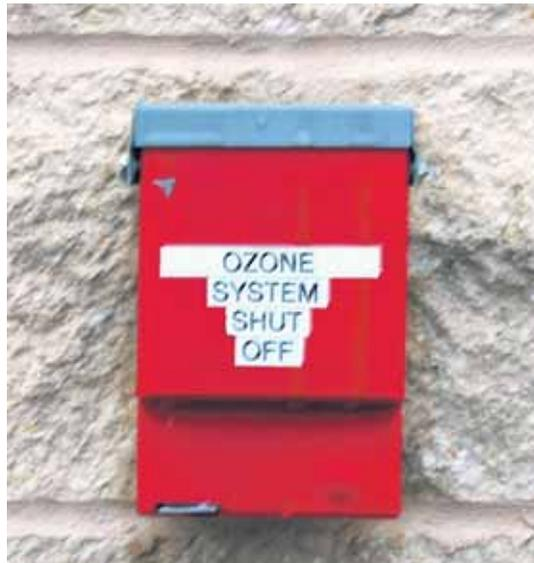
Ozone generator emergency shut-off should be located OUTSIDE the generator room!
