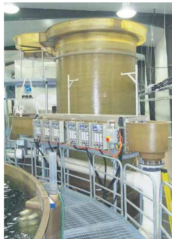
Cyclobio fluidized sand bio-filter at the Conservation Fund Freshwater Institute. The CO<sub>2</sub> stripper is stacked directly above a low head oxygenator and UV irradiation filter. The LHO unit is used to transfer an ozonated oxygen feed gas into the 4,800 l/min recirculating flow.
