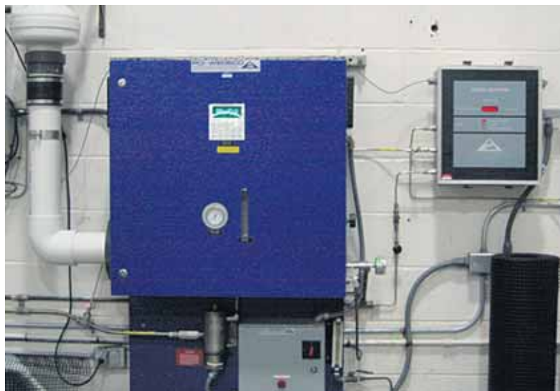
Ozone generator and high-concentration ozone gas monitor used at the Conservation Fund Freshwater Institute.
