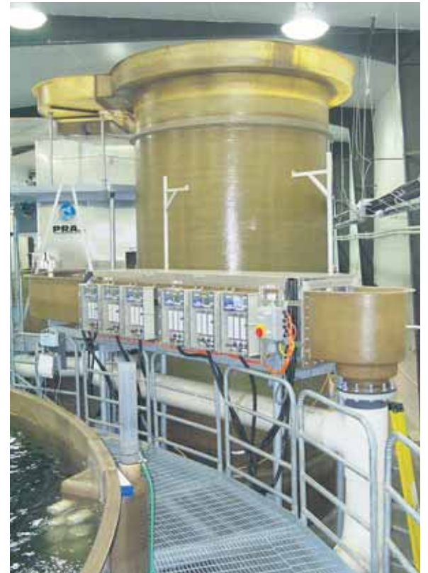
Cyclobio fluidized sand bio-filter at the Conservation Fund Freshwater Institute. The CO 2 stripper is stacked directly above a low head oxygenator and UV irradiation filter. The LHO unit is used to transfer an ozonated oxygen feed gas into the 4,800 l/min recirculating flow.
