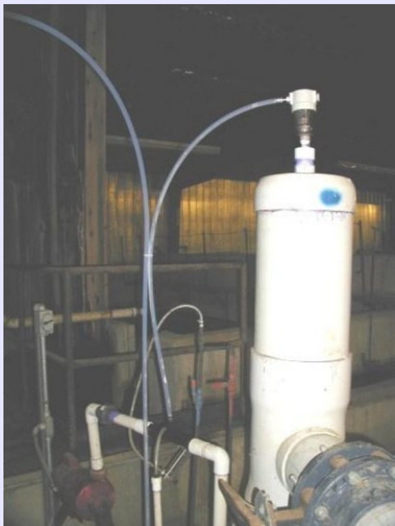
This air vent removes undissolved ozone gas for eventual reinjection into a separate water line at a Talapia fish farm.
